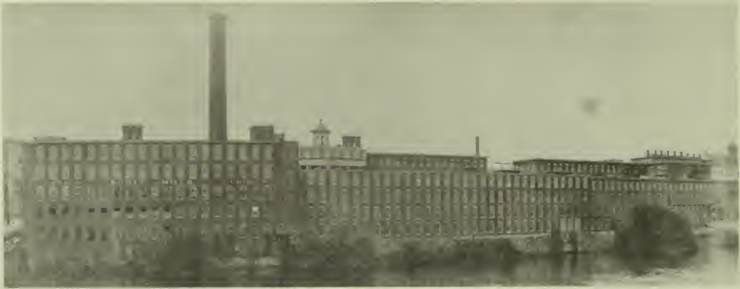
Figure 1. The windows are the dominant element of detail and decoration in the Boott Cotton Mills. Photo: Courtesy of the Center for Lowell History
